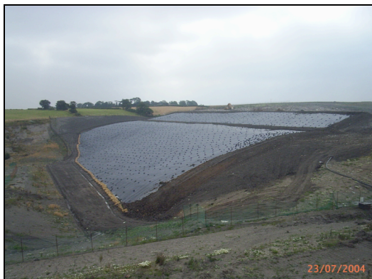
Photo 3: Completed capped cell
