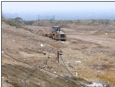
Photo 17: Unprotected leachate extraction point
