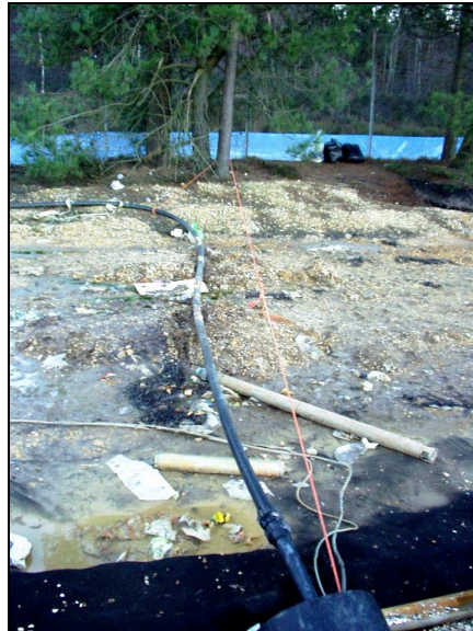
Photo 20: Open side riser
