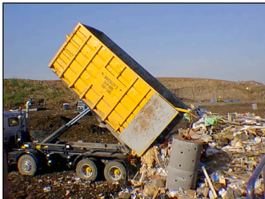
Photo 6: Depositing waste close to a leachate well
