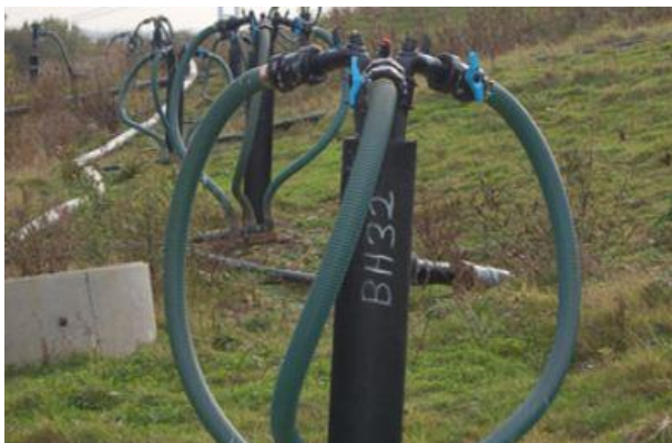
Multi-stage wells - flexible hose
