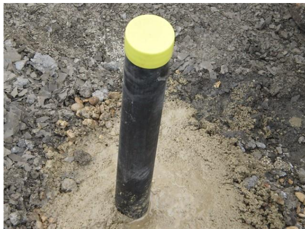
Good (well hydrated) bentonite seal
