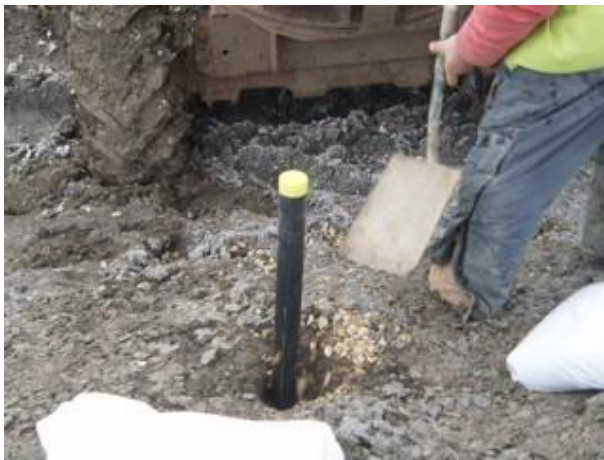
Gravel pack poured
