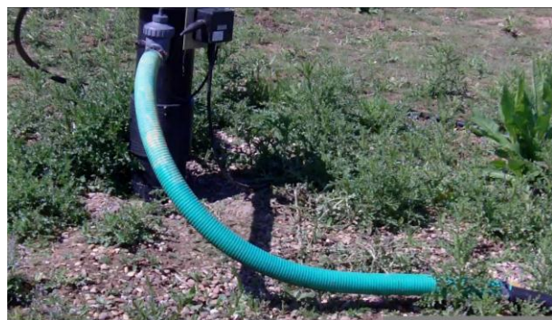
Flexible hose correct length connections
