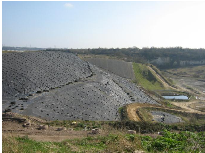
Figure 6.3: Good Waste Flank, with Temporary Capping
