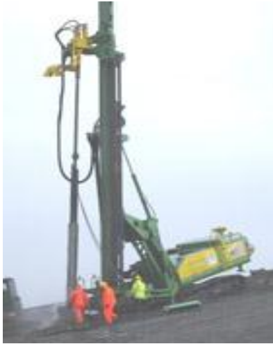
Figure 6.2: Drilling on a Slope
