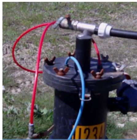
Figure 7.18: Air Pumped Wellhead
