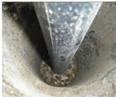
Figure 7.3: Gravel Pack Installation
