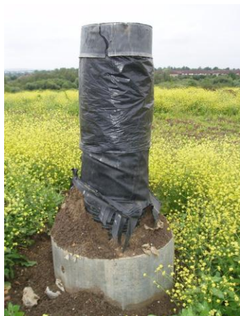
Leachate well - damaged seal
