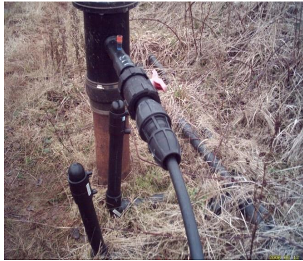
Well is connected without flexible hose
