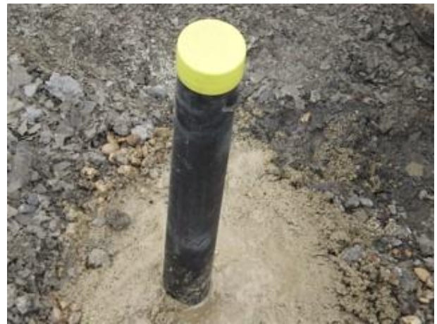
Bentonite seal poured
