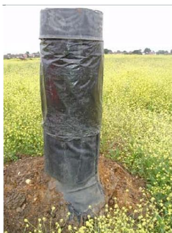
Leachate well - sealed after repair
